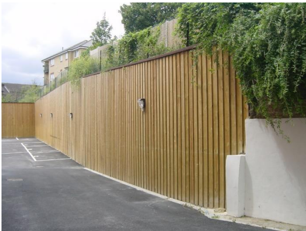
Photo 1. Completion with a Wooden Clad
