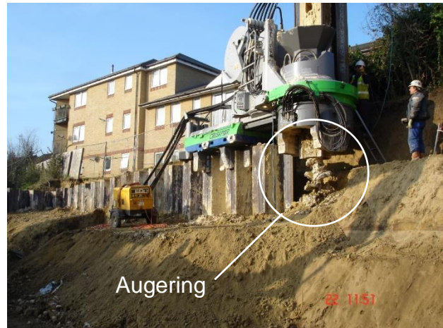
Photo 2. Piling Work in Progress
