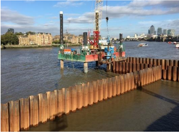
Photo 4. Press-in operation on water
