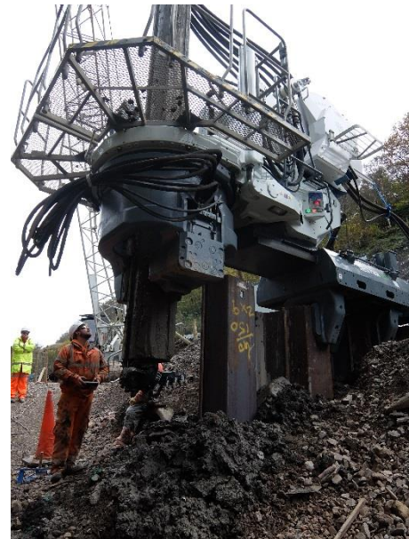
Photo 2. Piling on slope
