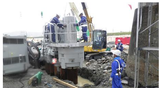
Fig. 9 View of the steel pipe pile press-in work
