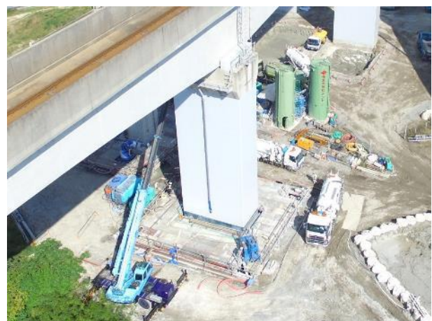
Photo 3. View of the soil improvement (outbound 2P)
