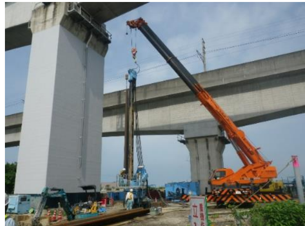
Photo 1. View of installing steel sheet piles (outbound 2P)
