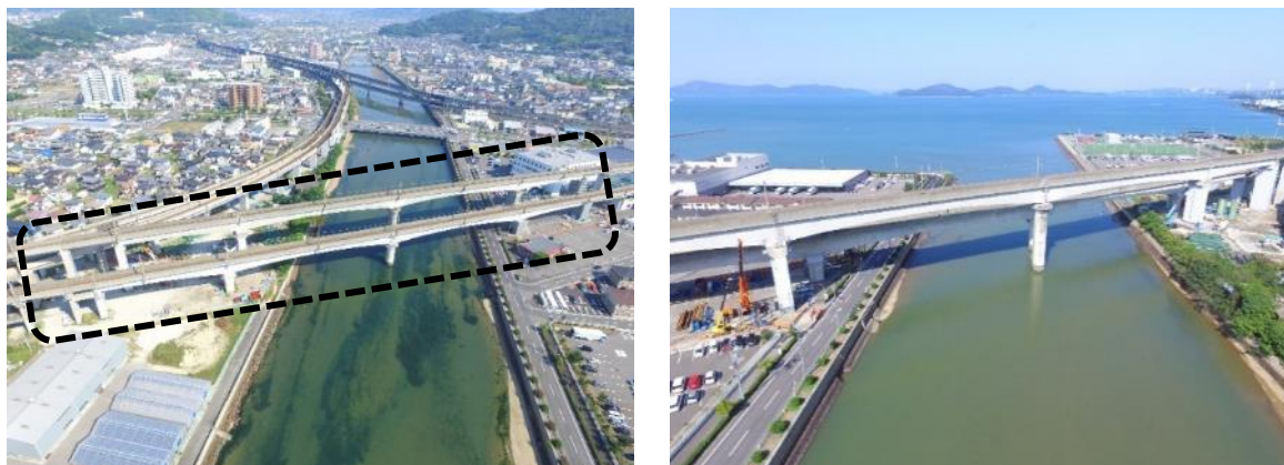
Fig. 2 Full view of Daisokugawa Bridge
