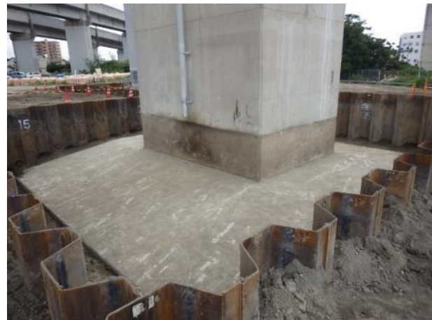
Photo 2. View of the installed steel sheet piles (inbound 2P)
