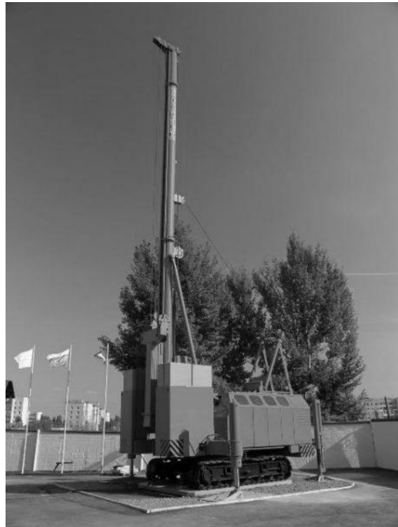
Photo 8. SVU-6 pile driver (Russia, Ukraine)
