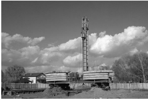
Photo 9. VIF pile driver (Ukraine)
