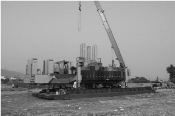
Photo 6. ZYB pile driver (China)
