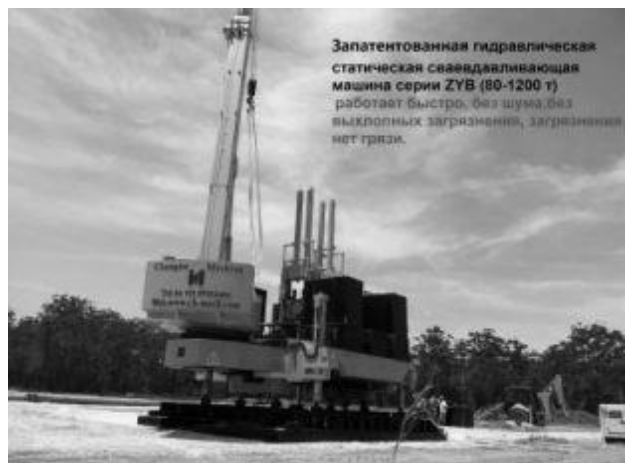
Photo 5. ZYB pile driver (China)
