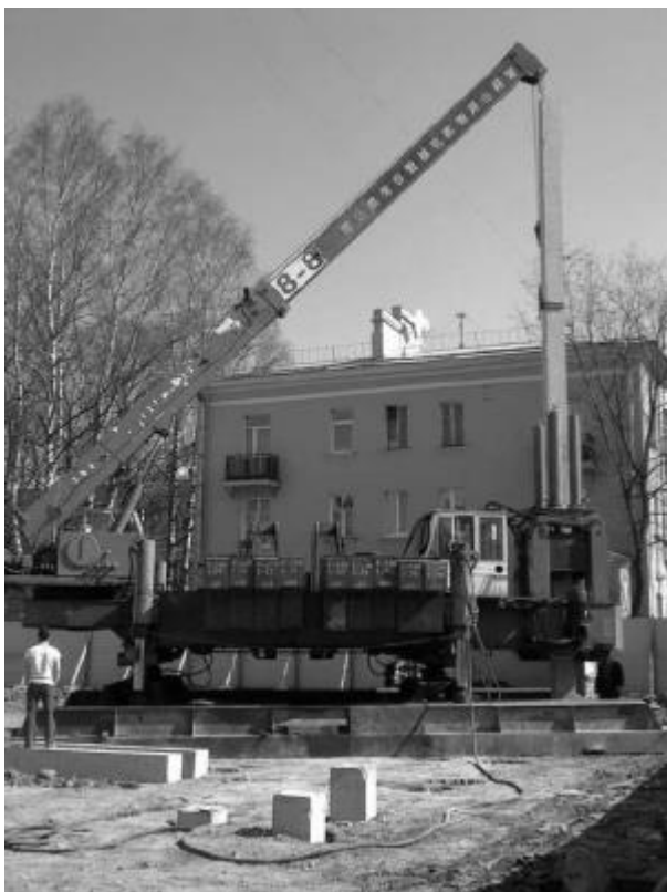
Photo 7. Starke pile driver (China)
