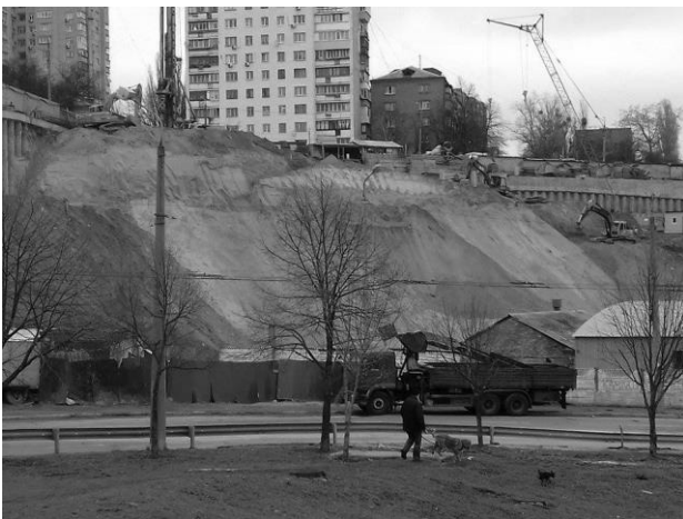
Photo 3. Landslide in Kyiv
