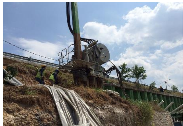
Fig. 3 Retaining structure construction for highway near Taman Jasmin Indah
