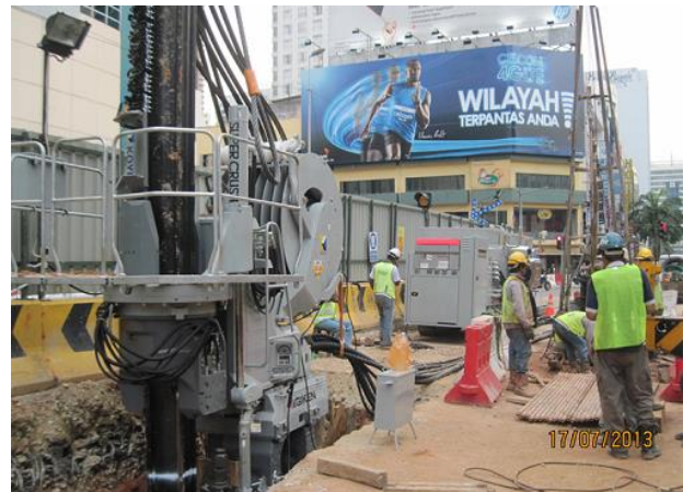
Fig. 2 Construction at Bukit Bintang MRT Station
