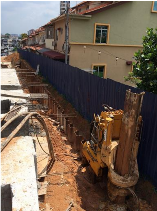
Fig. 5 Sheet pile installed for commercial development near residential area
