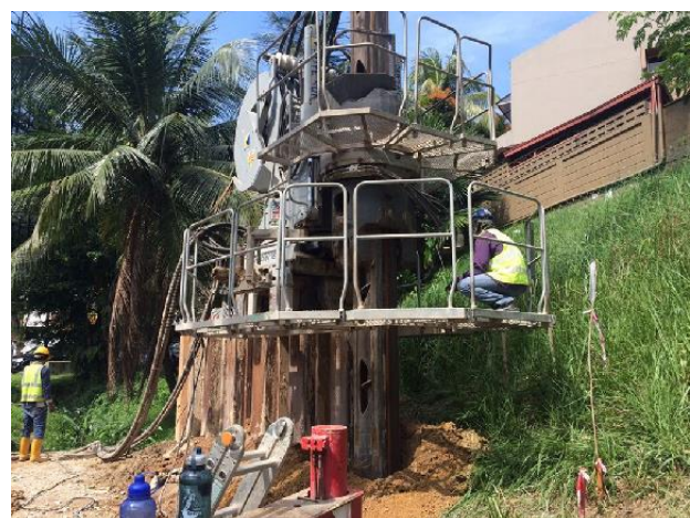
Fig. 4 Sheet pile installed by Super Crush Piler at Sprint Highway
