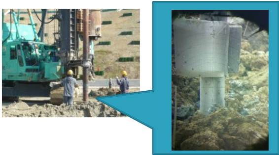
Fig. 11 PM Method, Stage 4, before final pile settlement
