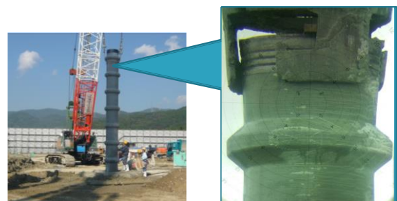
Fig. 10 PM Method, Stage 3, during pile installation
